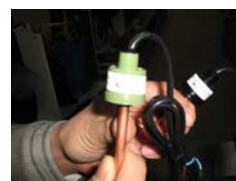
Figure 47: Pressostat de pression maximale.
