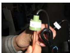
Figure 46: Pressostat de pression maximale.
